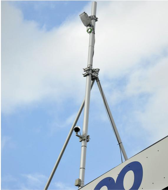
Figure 2: ZXY radio receiver mounted on antennas around the stadium.
